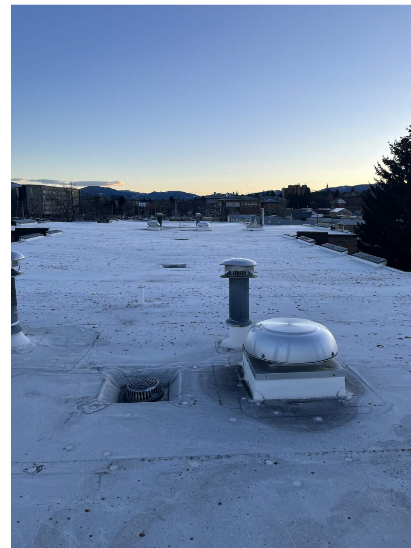
EXISTING ROOF WITH DRAIN, BOILER VENT, AND RELIEF VENT., TYPICAL CONDITION.
