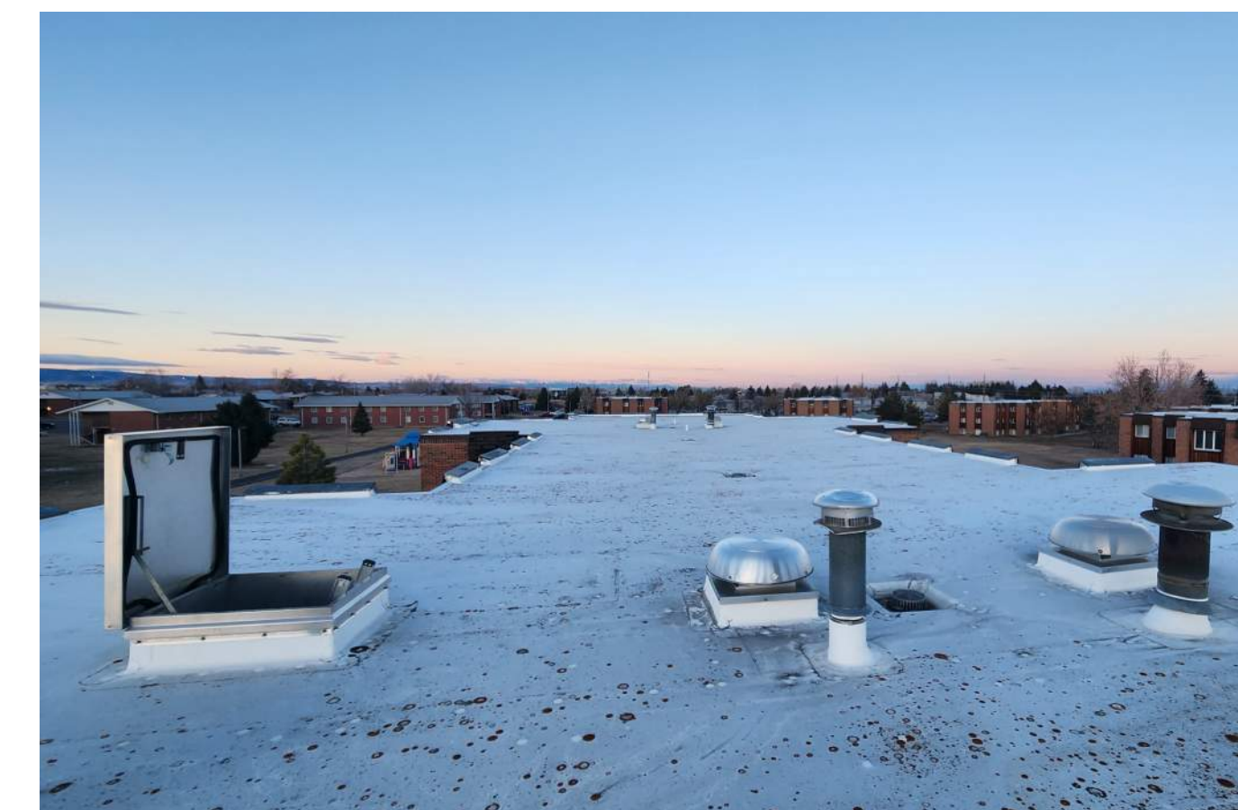
EXISTING ROOF HATCH, TYPICAL CONDITION.
