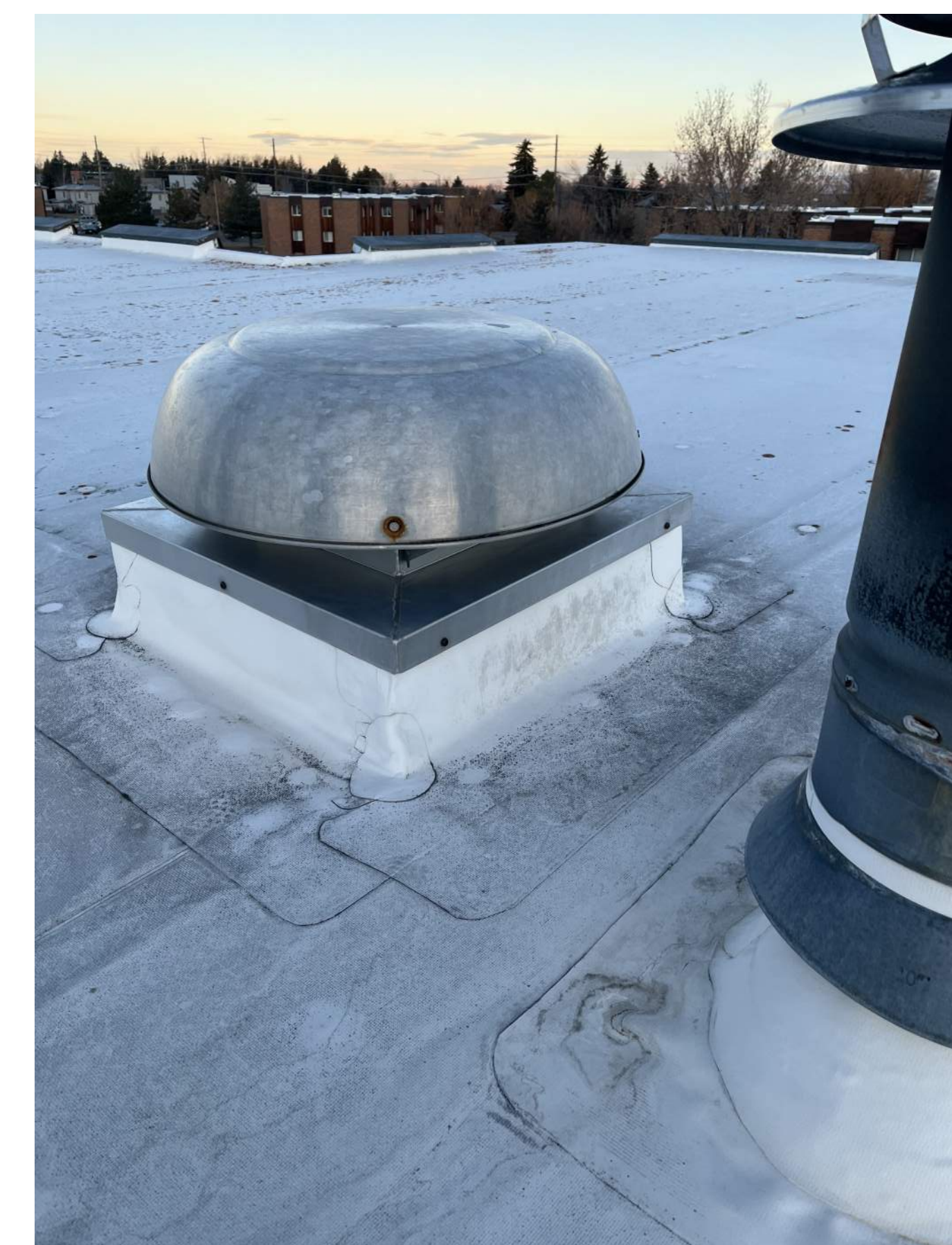
EXISTING RELIEF VENT, TYPICAL CONDITION.
