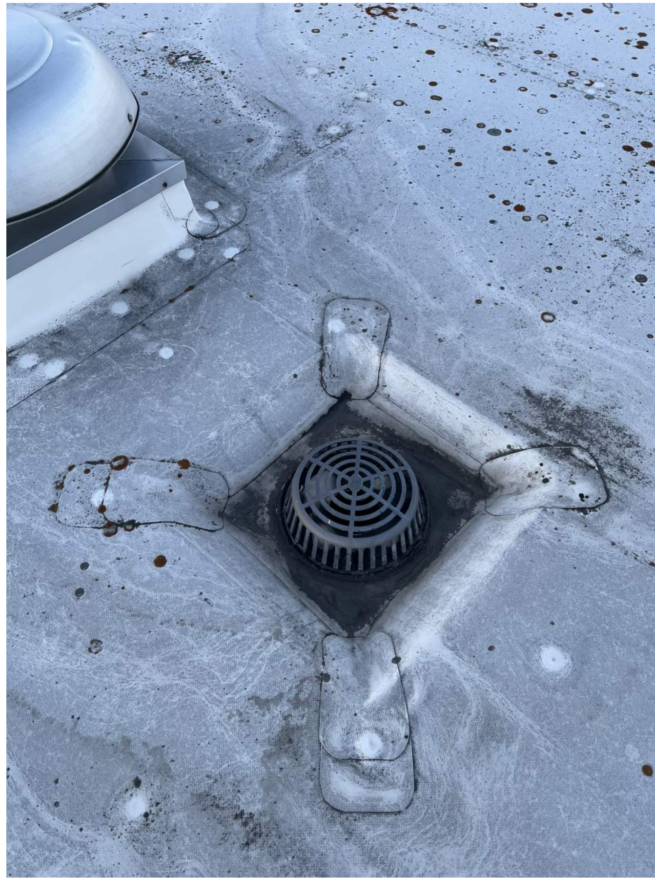
EXISTING ROOF DRAIN, TYPICAL CONDITION.
