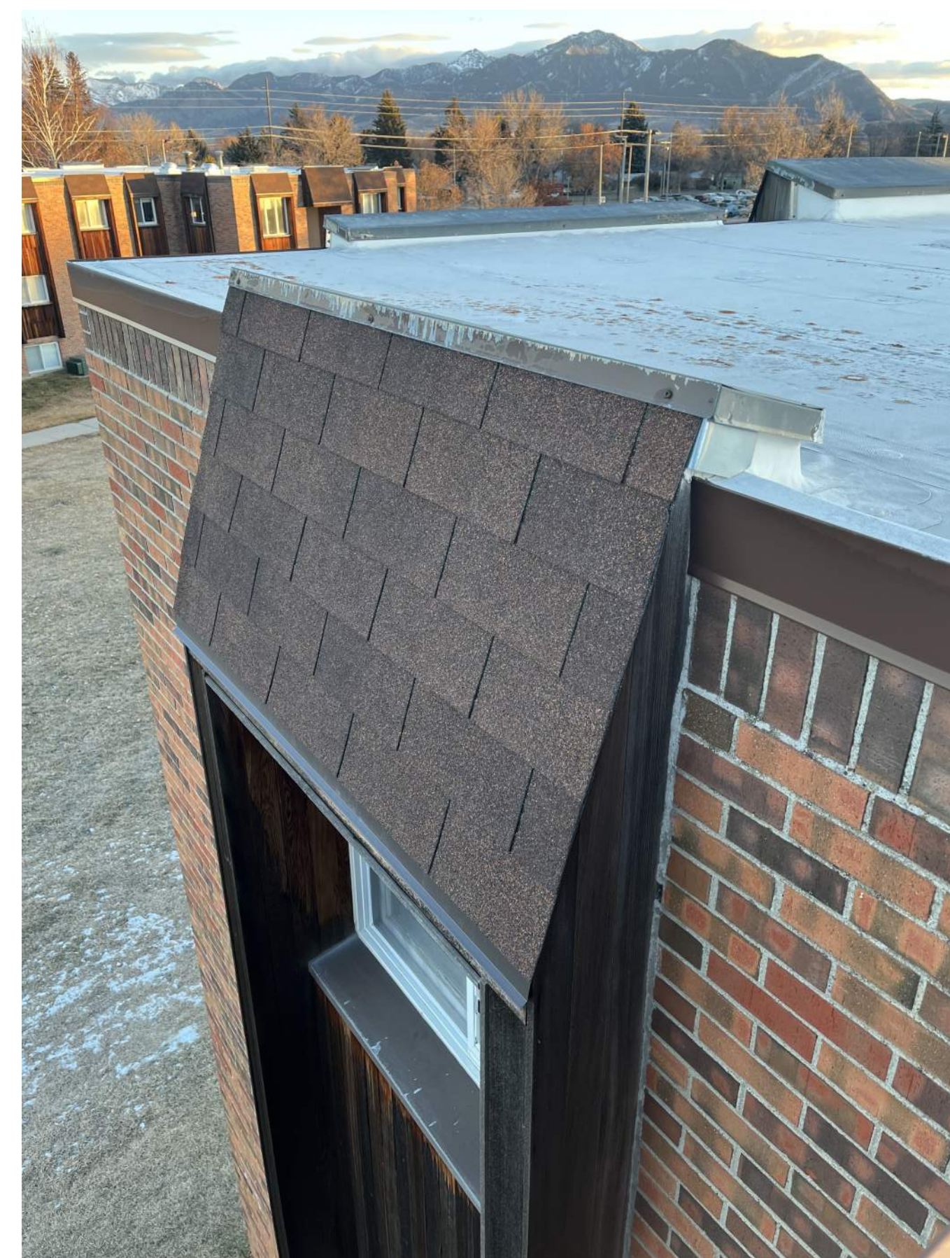
EXISTING DECORATIVE ROOF, TYPICAL CONDITION.
