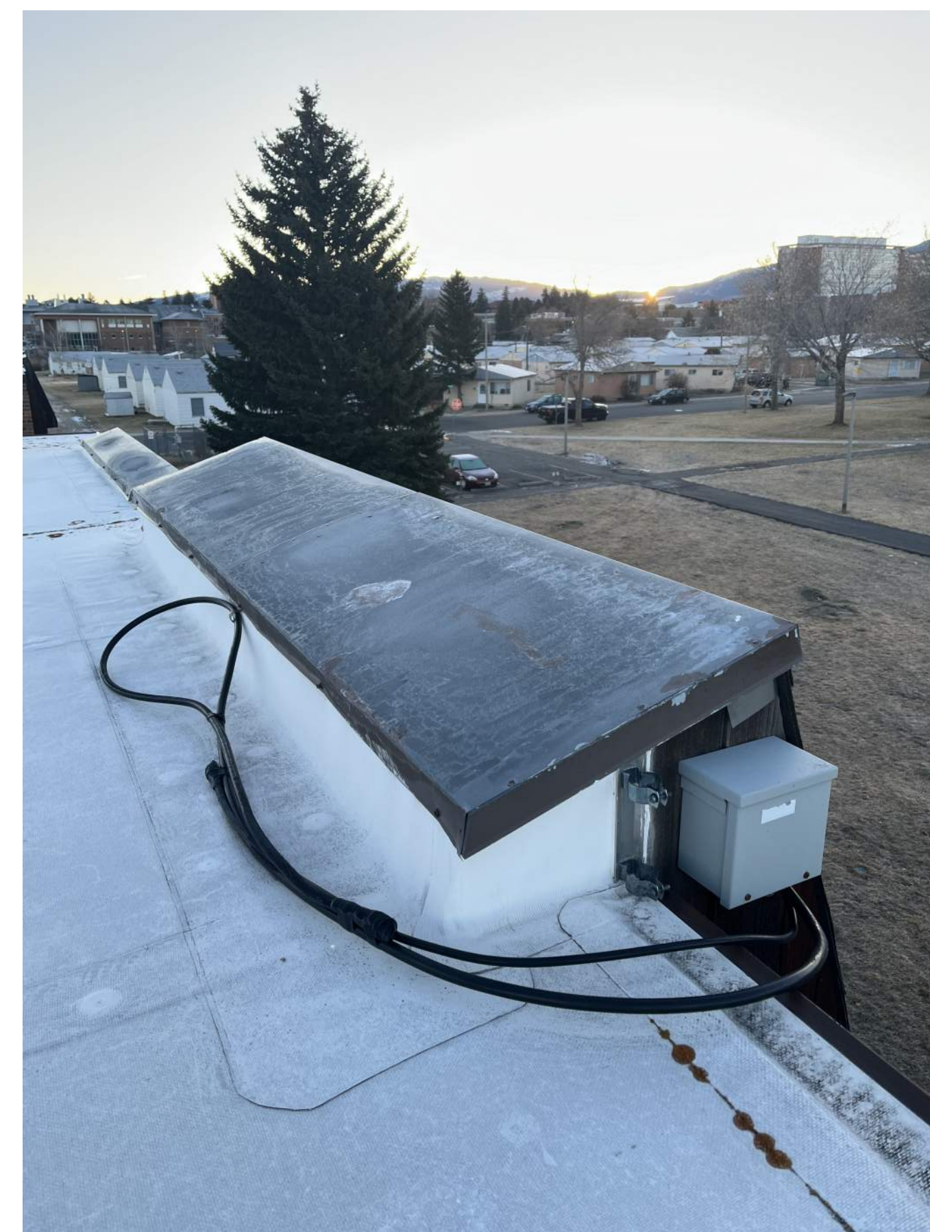
EXISTING COPING EDGE AT DECORATIVE ROOF LOCATION, TYPICAL CONDITION.
